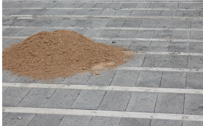
Infilled floor with grout
