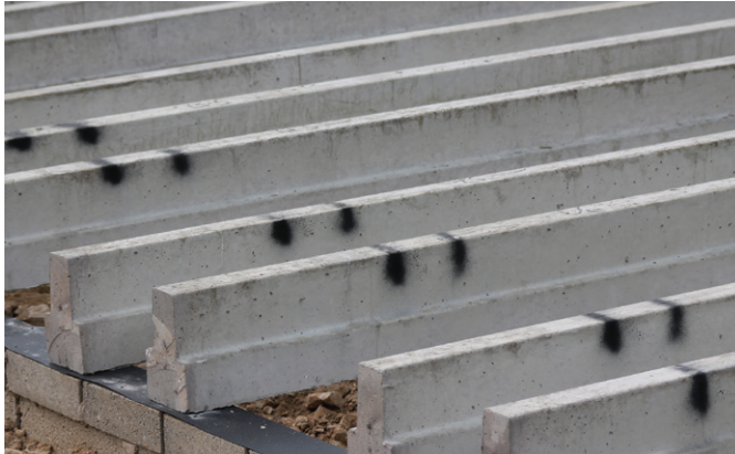
Beams in place
